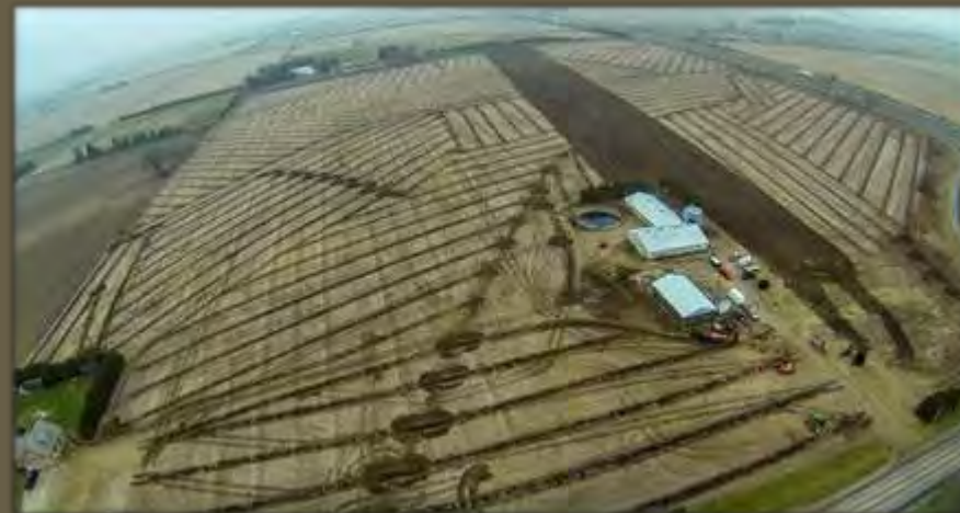
Extensive tile drainage
