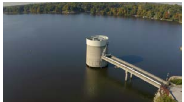
Drinking water intake at Eagle Creek Reservoir Photo credit: 12 Stars Media
