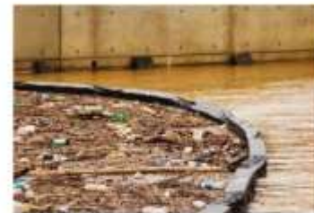
Boom captures litter and other debris carried by stormwater.
