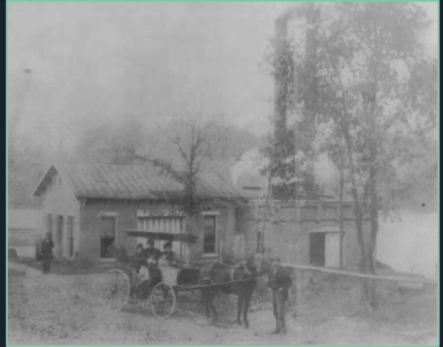
Bloomington's first waterworks plant (Twin Lakes)
