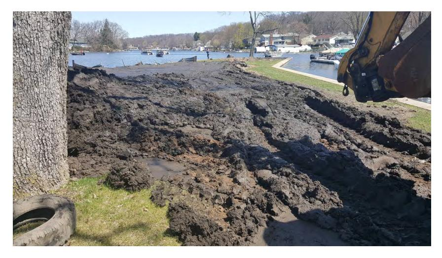
Material is very sloppy and runny. Contains over 50% water. Removing enough water to make the material manageable is difficult and costly.
