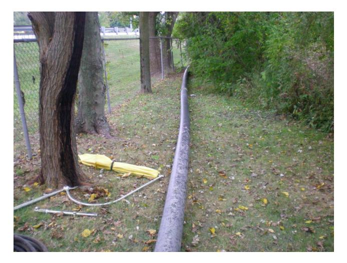
The pump sends a slurry of roughly 25% material and 75% water through a 6" diameter plastic pipe to an onshore disposal area.
