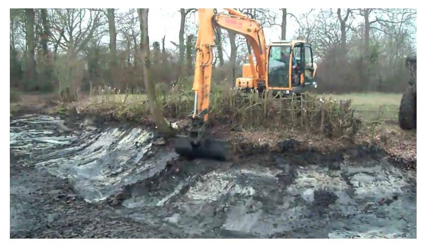
For small ponds a conventional excavator or long stick excavator can be used from shore to remove the sediment and load directly in to trucks
