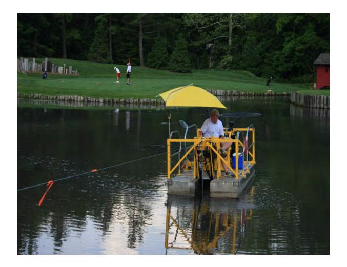
A floating barge is placed in the water and cables are used to control the lateral movement
