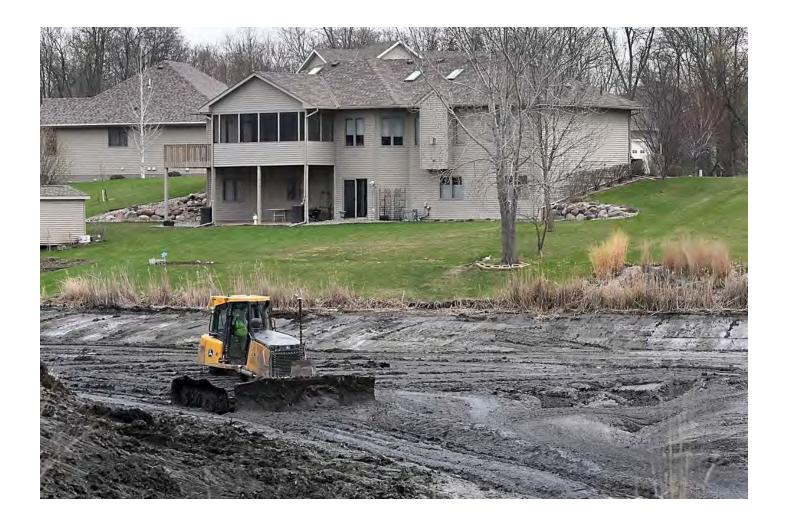
Larger ponds require equipment in the pond to push the material to a loading point near the edge of the pond.
