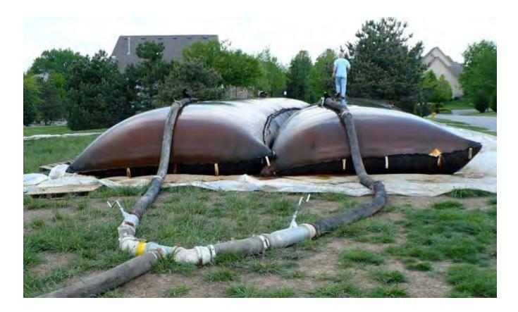
Geotextile Tubes – Large fabric containers (typically 30' to 50' wide, 50' to 100' long and up to 10' tall) made from heavy duty woven geotextile fabric
