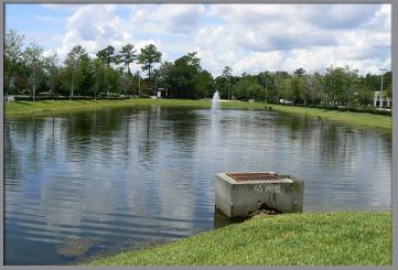
A detention pond and outlet control structure
