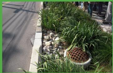
This roadside swale infiltrates water but also has an overflow drain to capture water during larger storms.
