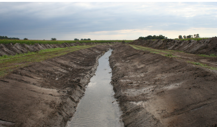
Excavated section of two-stage on the Shatto Ditch project before seeding
