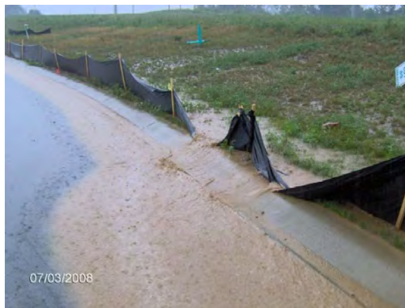
Figure 4-1: Poorly installed silt fencing
