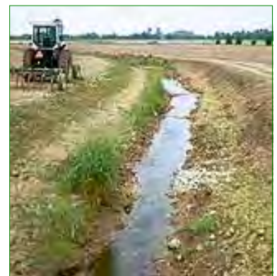
Newly constructed 2-stage ditch
