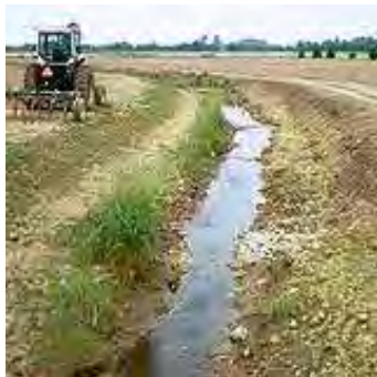
Newly Constructed 2-Stage Ditch
