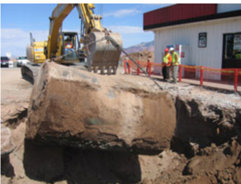
Removal of an underground storage tank
