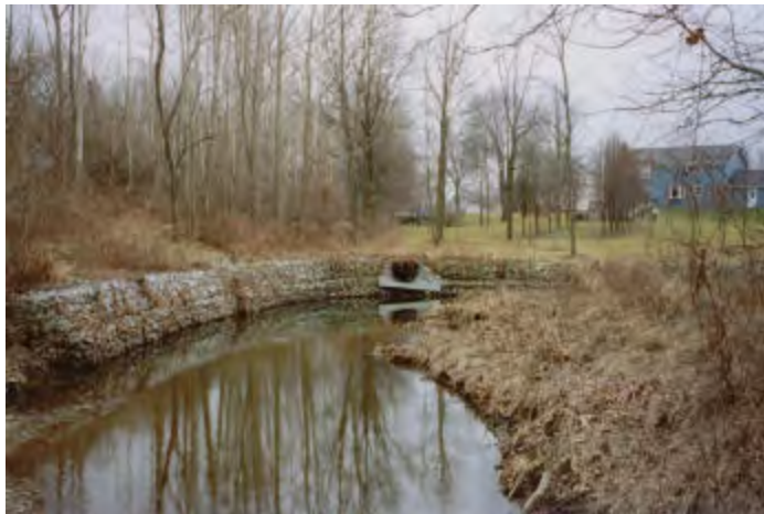
Example of Gabion channel bank stabilization on Cool Creek near Underwood Court in City of Carmel
