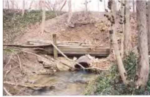
Culvert Pipe Collapse and Erosion
