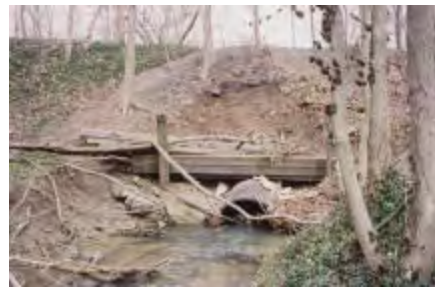
Upstream end of existing 48-inch culvert outlet (note pipe section has fallen into creek and embankment is eroding above culvert)
