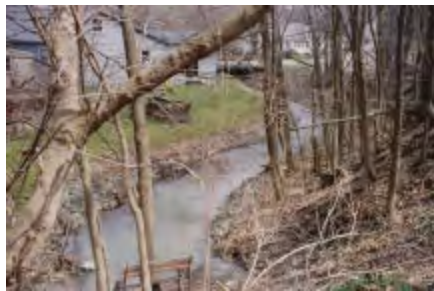
Downstream of 48-inch culvert outlet (note how existing outlet is at a channel bend and is subject to erosion)
