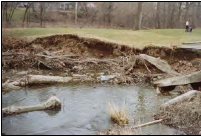
Cool Creek in Brookshire Golf Course Severe Bank Erosion, Cart Path Fallen into Creek
