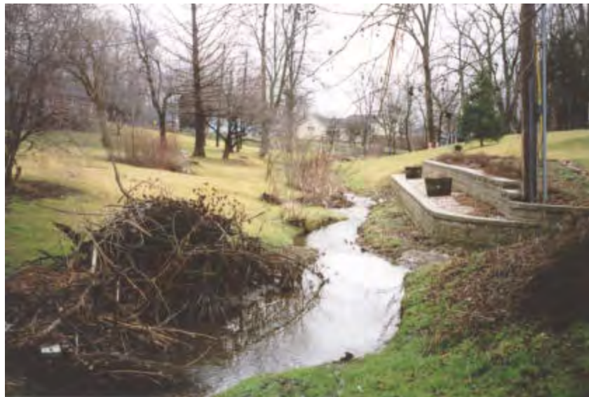
Construction near channel (right side of photo) constricts flood waters and promotes downstream erosion. Landscape debris (left side of photo) prevents the efficient flow of water and traps additional debris, creating a dam.
