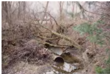
Breach in abandoned railroad embankment (note deteriorated CMP, pipe in foreground appears to be a bucket or rubbish container)
