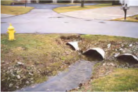
Culvert in Need of Sediment Cleanout
